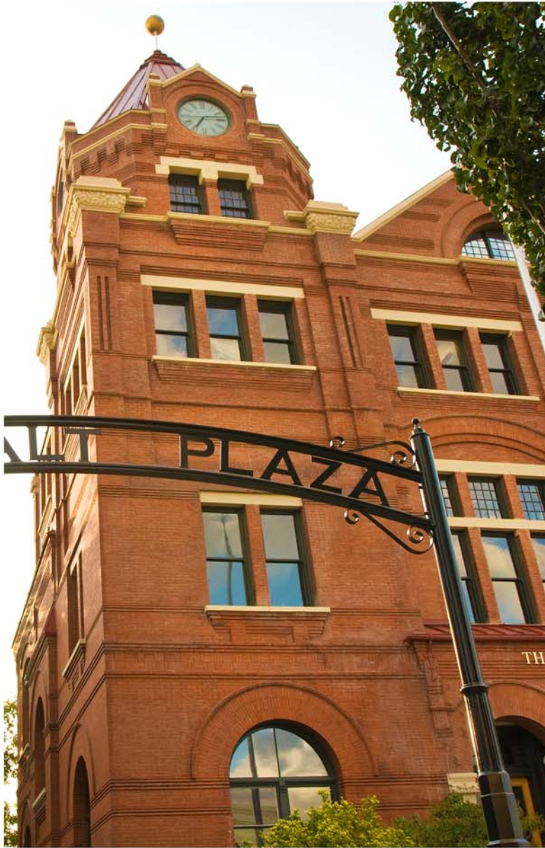
Downtown Heart} Carson City's iconic Laxalt clock tower immediately borders project area.
